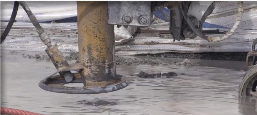
Water used for hydrodemolition operations can be collected on-site, treated, and then recycled back into the system.
